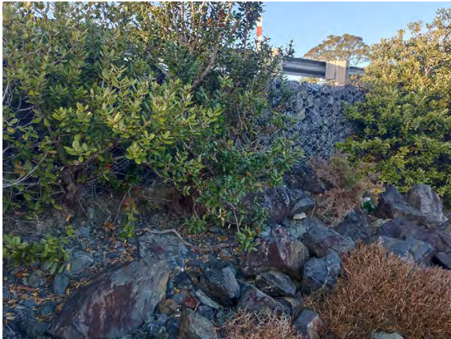
Photograph 2.2b: Gabion and rock riprap to causeway
